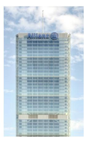
With its 50 floors, the 207 m high tower within CityLife area is one of the tallest buildings in Italy. The base is narrow and long, thus accelerating the building's verticality. A convex glass modular system supported by 3 steel struts reduces wind and seismic loads.
