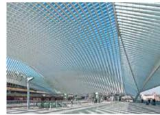
This high-speed railway station is one of the most important hubs in Belgium. It is made of steel, glass and white concrete. It includes a monumental arch, 160 m long and 32 m heigh. It has 9 tracks and 5 platforms and is used by 15,000 people every day.
