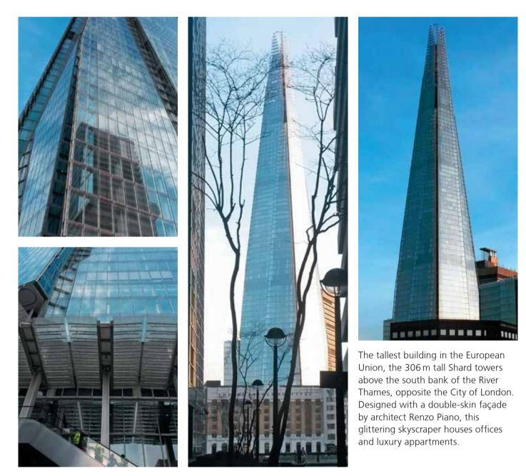
For the external wall, 40,000 m<sup>2</sup> of ipasol Bright White solar control glass incorporated in a laminated assembly with extraclear glass were supplied, 40,000 m<sup>2</sup> of iplus super-insulating glass integrated in double-glazing incorporating laminated extra-clear glass. The additional 12,000 m<sup>2</sup> of ipasol Neutral and iplus, used, respectively, for the complex double-glazing in the building's corners and ground floor.
